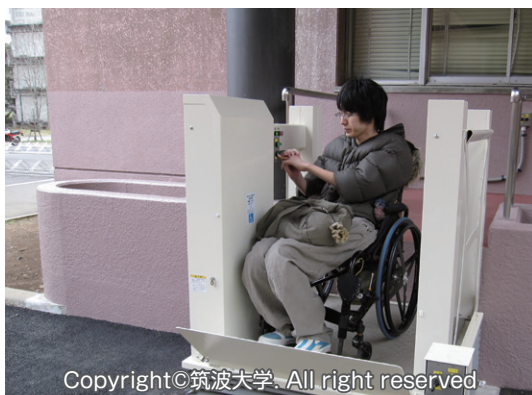
Copyright©筑波大学. All right reserved. (車椅子用昇降機)
