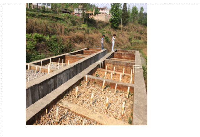
貴州省貴陽市鉞山排水処理試験場/The acid mine drainage (AMD) passive treatment system experimental station, Guiyang, Guizhou Province.
