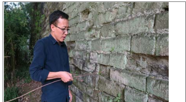
南京城壁調査/Survey on Nanjing city wall
