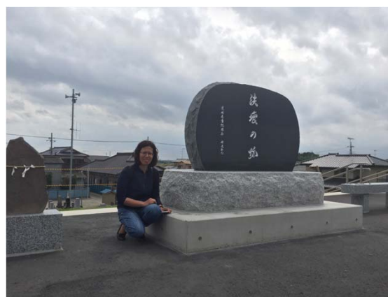
2015年に被災後復旧した鬼怒川堤防視察記念 (On-site inspection of the remediation from flood damage in Kuni-river dyke in Joso City)
